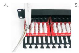
Use the LSA impact tool to punch and con- Use the cable tie to manage these cables, nect the wires on the IDC.
