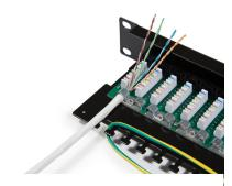
Follow the IDC colour-code for T568A or T568B wiring and set pairs into proper position.
